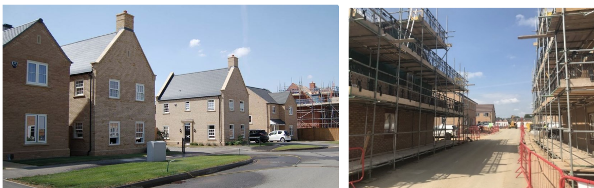
Fig 15 and 16: Medesham Homes completions and live on-site delivery
